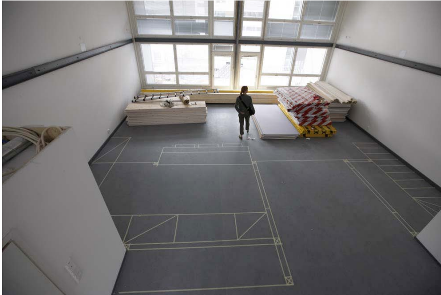
A typical “empty” unit with the dwelling unit floor plan drawn on the floor. The two bathrooms installed as part of the base building are visible in the foreground, one on each side of the space.
