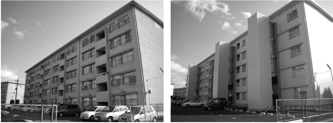
Figure 5 Building Before and After Elevator Towers Addition
