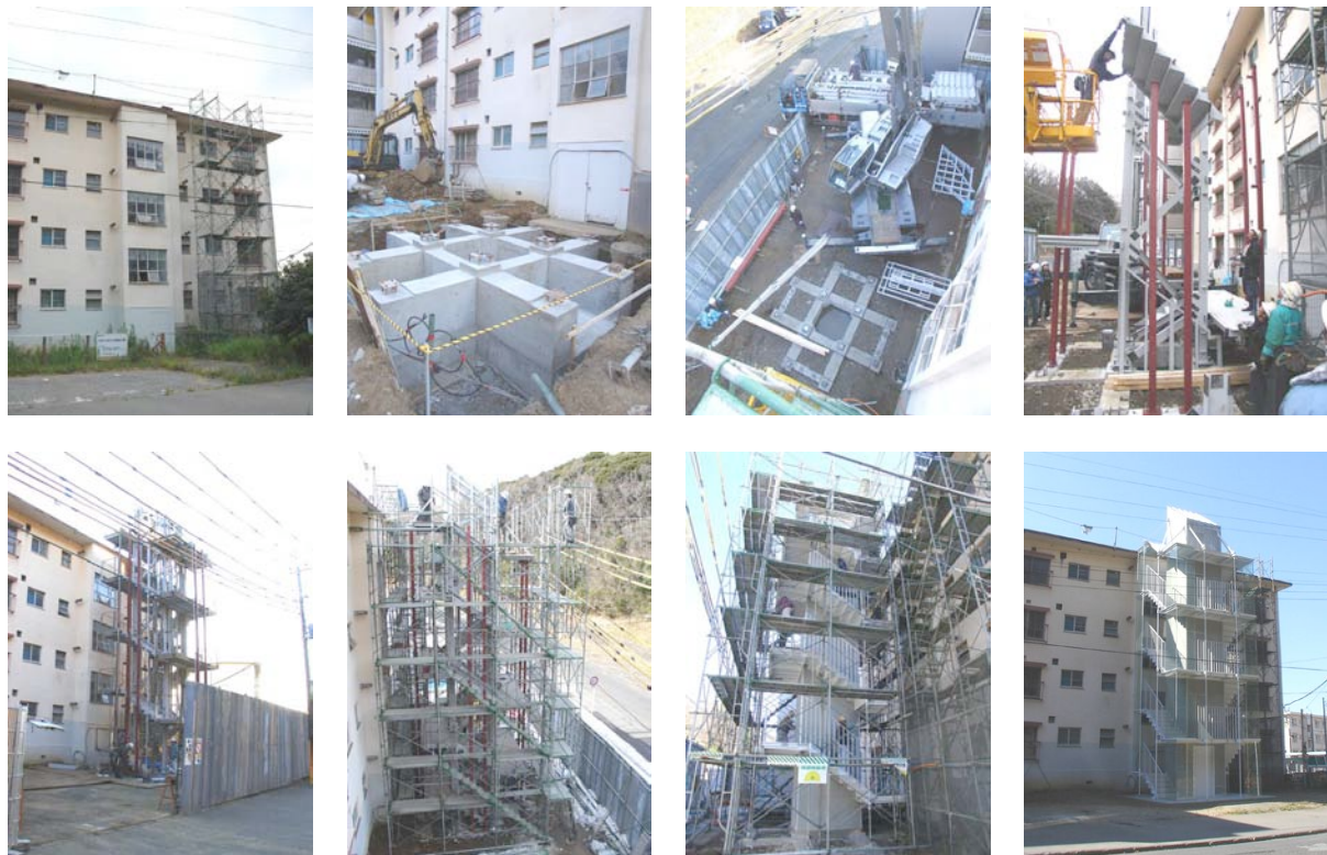
Figure 4. Process photographs of construction site
