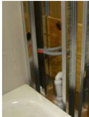
Figure 9: Pipes in partition wall (left); Figure 10, 11: Pipes between double walls (middle and right)
