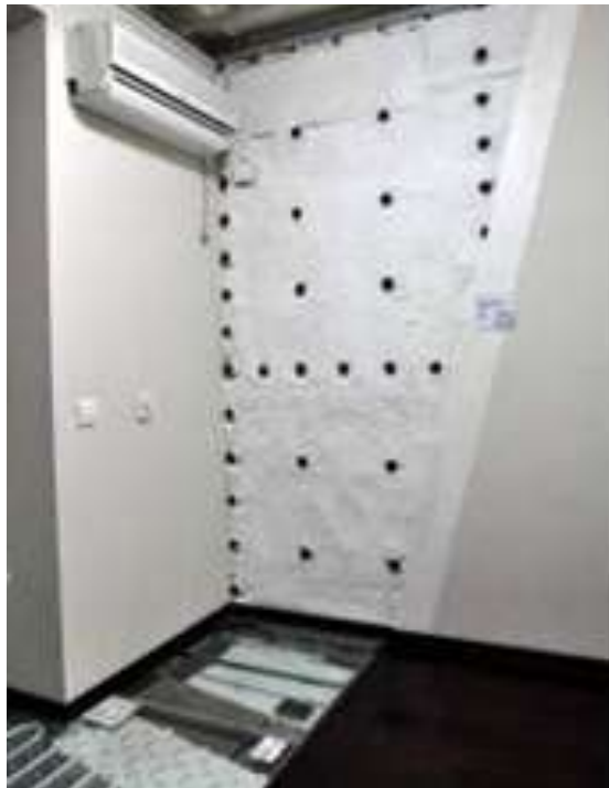
Figure 5: Inner heat preservation system. Resource: CNERCHS
