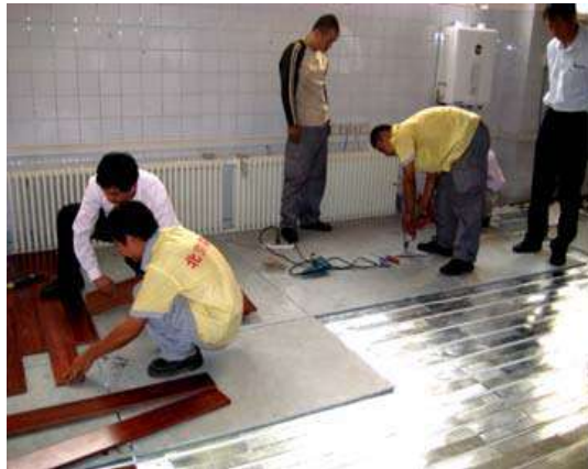
Figure 4: Construction sample of dry ground heating floor
