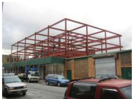
Figure 8: Two-Story Steel Frame on Base of existing building
