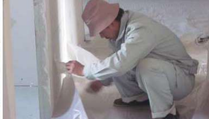
Figure 11: Laying protective covering on the floor
