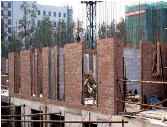
Figure 6: Construction sample of fair-faced concrete block
