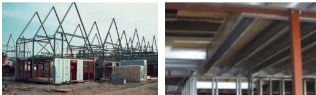
Figure 5: the Corus metal floor system makes the adaptability of services and cabling possible after realization of the homes.
