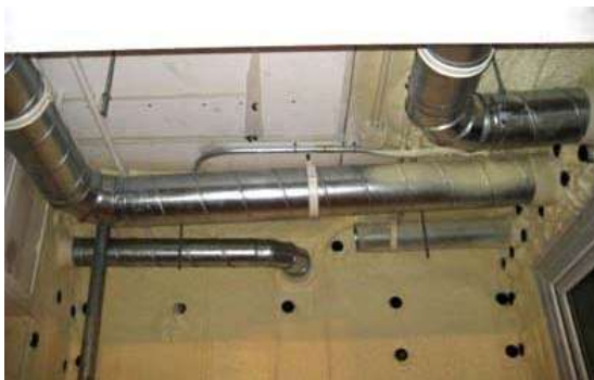
Figure 14: Reserved pipeline holes sample that is connected with the outside wall
