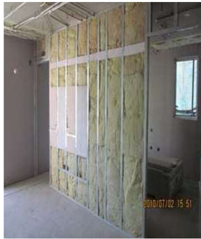
(b) Light steel keel plasterboard internal partition wall
