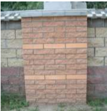
Figure 5: wall constructed using 90 mm high blocks
