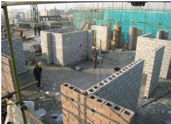
Figure 10: Joint connection of the exterior and interior walls
