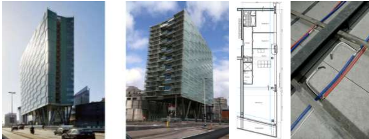
Figure 7: La Fenêtre case with 115 homes spread across 16 floors; the Infra+ metal floor system, with an extra concrete finishing layer against sound problems which prevented most of the future adaptability
